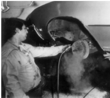
Figure 1: Visual of how much asbestos containing dust from friction linings becomes airborne when cleaning with compressed air. Source: Rohl et al. 1976 (Figure 4).
